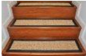
Standwoven Bamboo installed.
